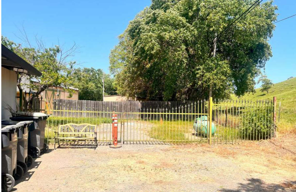
Photo 13: Existing Septic Leachfield located behind the Filling Station
