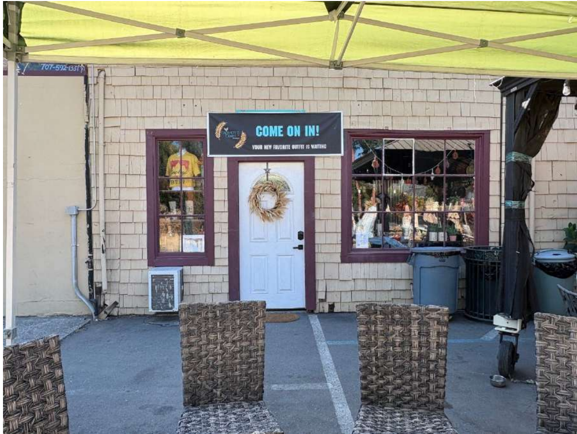
Photo 9: Existing Farmer's Closet façade
