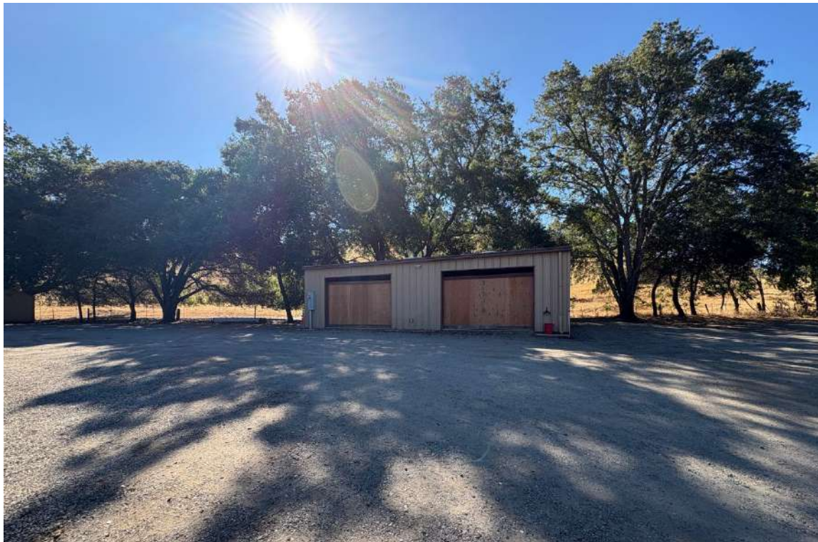
Photo 14: The vacant 1,111-sf steel building on Clayton Road to be repurposed for the Wild Oak Wellness (WOW) business.
